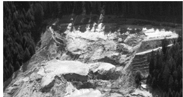
Figure 3. The Stava embankment after the failure ([26]).
