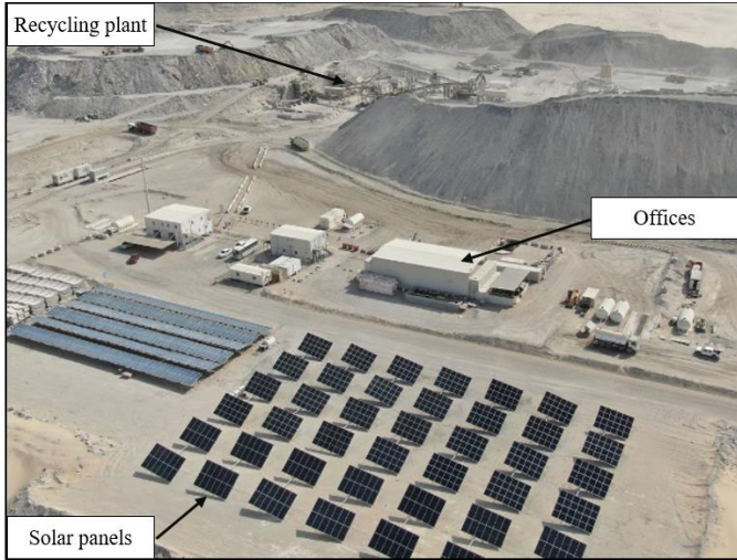
Figure 2. An aerial view of Al Dhafra recycling plant [23].
