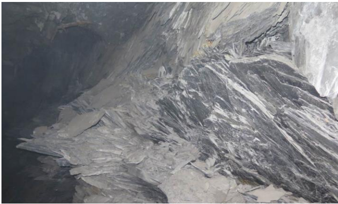
Figure 13. Creep buckling of the pelites at some galleries in Draa Sfar mine
