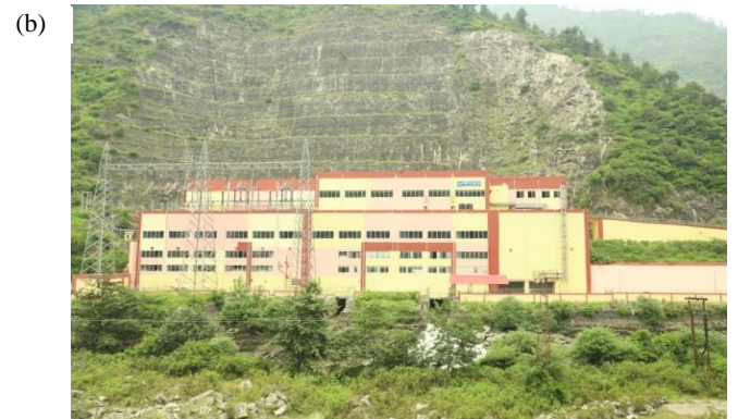
Figure 1. (a) Layout plan of Parbati hydroelectric project-II (b) View of surface powerhouse of Parbati hydroelectric project-II, NHPC [7]
