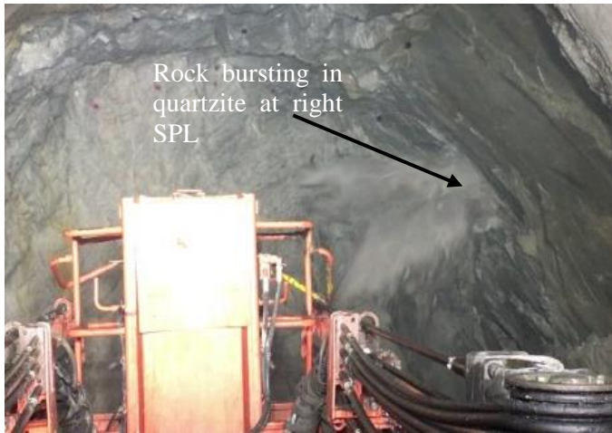
Figure 21. Rock bursting in right springline (SPL) area of HRT
