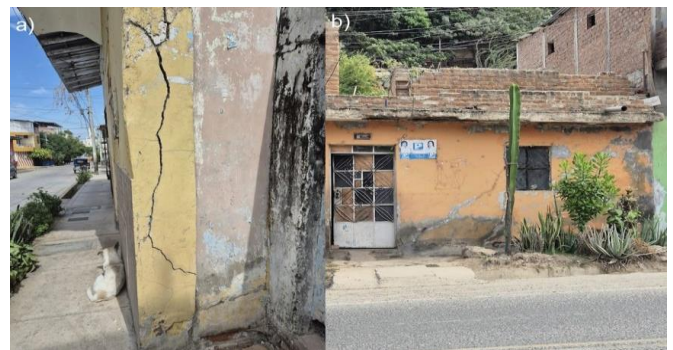
Figure 1. Structures damaged by expansive clays in Sullana.
