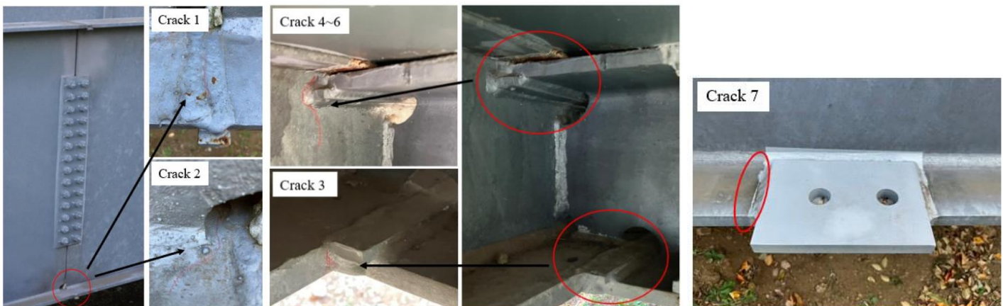
Figure 3. Simulated cracks drawn on structural joints of the test bridge.
